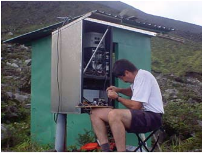
Figure A6.2. One of IRIS's long-term instrument loans was to permanently improve monitoring on the Nicoya Peninsula, Costa Rica, by helping Universidad Nacional to re-occupy vaults that were constructed for PASSCAL experiments. Here, Victor Gonzalez of UNA services a station that part of a cooperative, multi-disciplinary project with the University of California, Santa Cruz, to monitor Arenal Volcano. Other instruments were loaned to AfricaArray, the University of Bangladesh, the Kyrgyzstan Seismic Network, and Instituto Nacional de Prevención Sísmica, Argentina.
