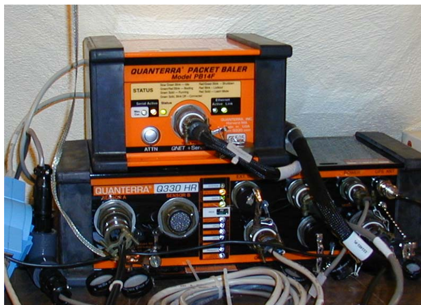
Figure 3.4.1 Q330HR Testing in ASL Tunnel
