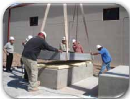
Figure A2.4. (left) Completed PIC external sensor vault building. (right) Crane lowering granite slab into place on one of the two piers during construction. Photos provided by Bruce Beaudoin.
