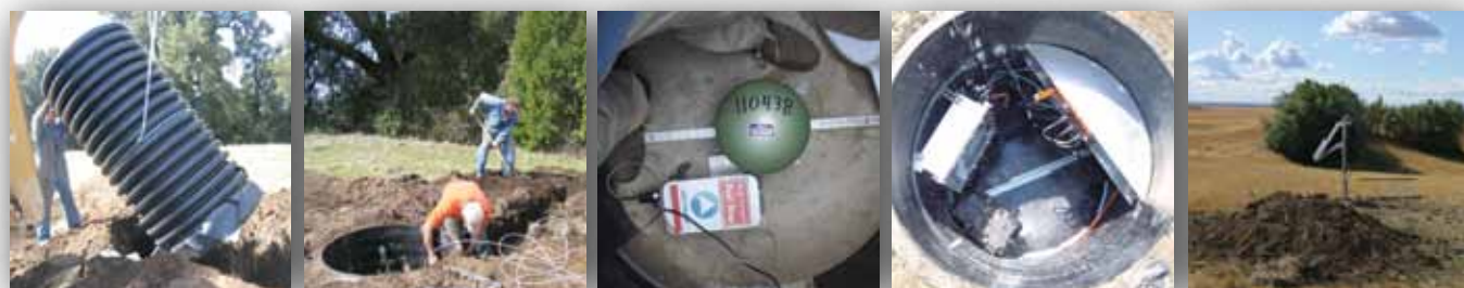
Figure A5.2. Installation of a Transportable Array station (left panels), instrumentation (middle and middle right panels), and completed station (right panel). The vault is under the mound of dirt in the foreground.
