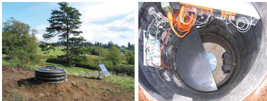
Figure 2.3. A typical Transportable Array station showing the relationship of the equipment inside the enclosure and the solar panel.
