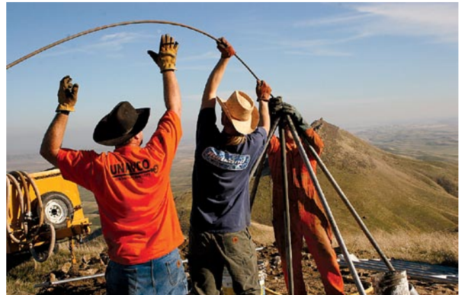
Figure 1.4. UNAVCO personnel installing a deep-drilled braced CGPS monument at Flat Top Peak in Southern California.
