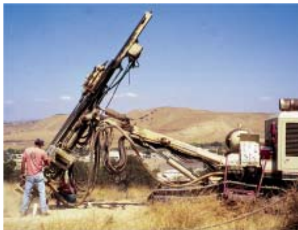
Figure II-2.3. Installation of station CRBT in the SCIGN network.
