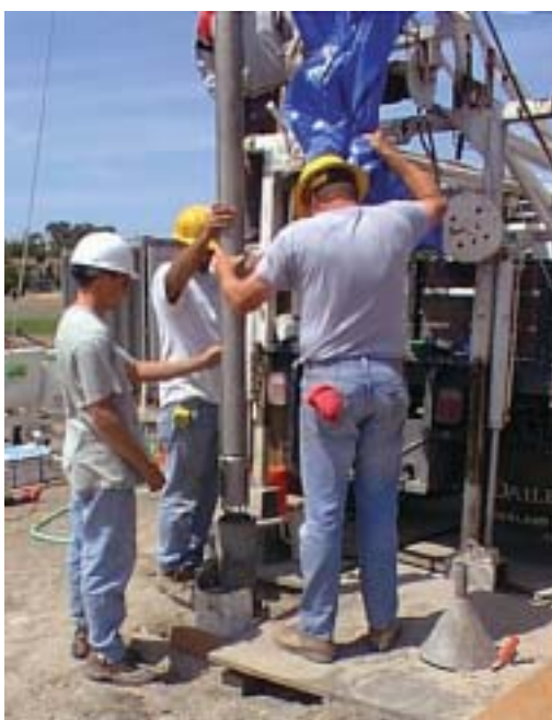
Figure II-22.14. Installation of a Gladwin Tensor Strainmeter instrument.
