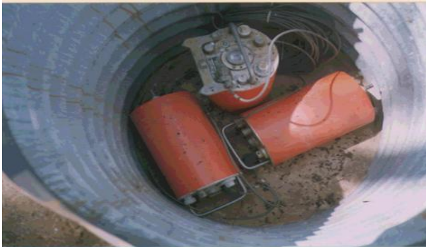
S-13 Short Period Seismometer in a Vault at Shai Hills .
